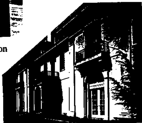
Figure 8: Oldfields Estate House
