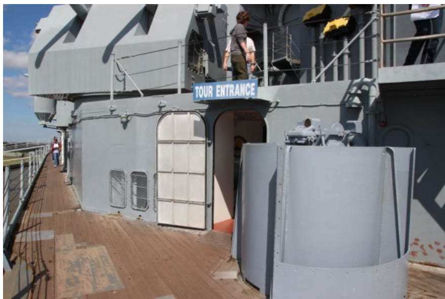
Above-Figure 8: Entrance to main exhibit hall, notice rust at bottom right and patches to deck on bottom left. Below-Figure 9: Two of the display cases in the main exhibit hall.
