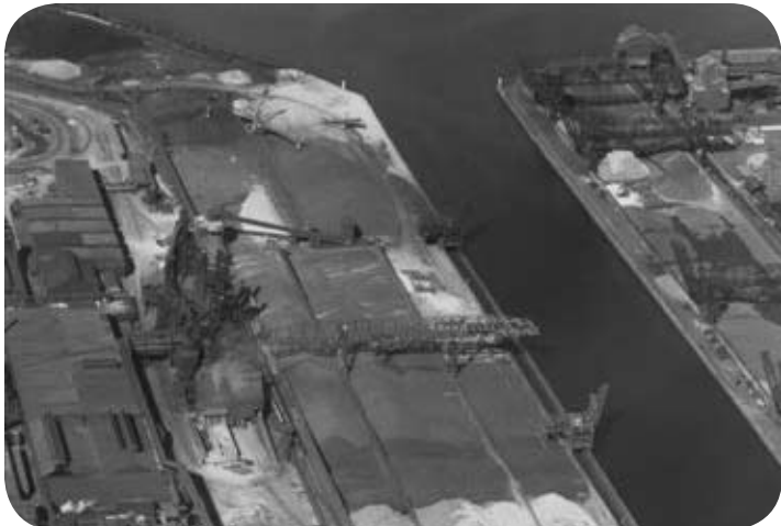
27. NORTH SLIP AND ORE WALLS (Photo by Okrent Associates, provided by Pamela Austin, McCaffery Interests)
