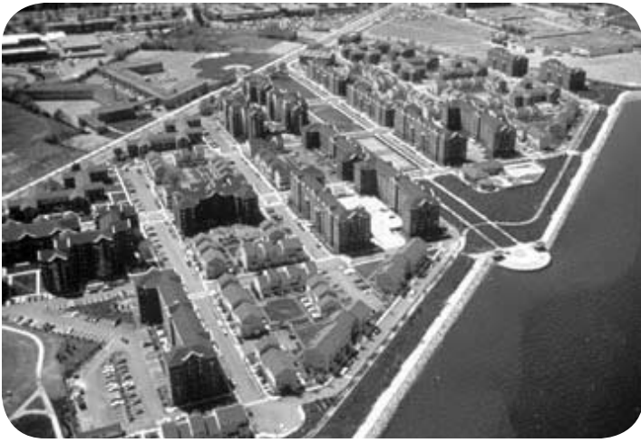
5. HARBOR POINT Aerial view of the development with its focus on establishing the waterfront as a positive space for the community. (Photo by Goody & Clancy)
