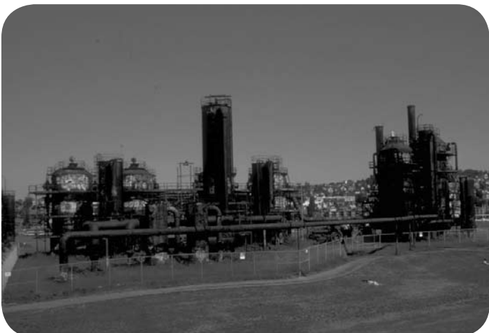
4. GASWORKS PARK Historic structures as Richard Haag deemed "sacred to the site." (Photo by Richard Haag Associates)
