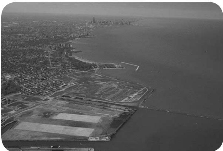
28. SOUTH WORKS SITE AFTER BUILDING REMOVAL (Photo by Okrent Associates, provided by Pamela Austin, McCaffery Interests)
