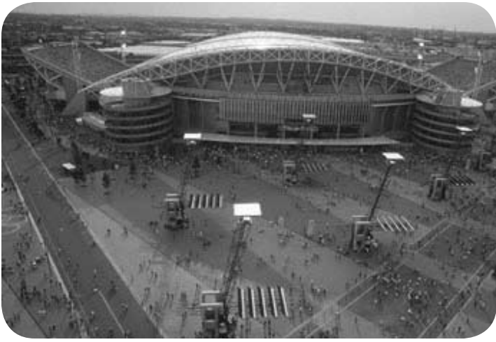
13. SYDNEY OLYMPIC PARK Olympic plaza with porous paving which funnels water to a trench system leading to a constructed wetland. (Photo by Hargreaves Associates)
