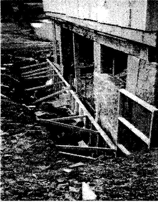
Above: Formwork has been built along the east in preparation for pouring the foundations.
