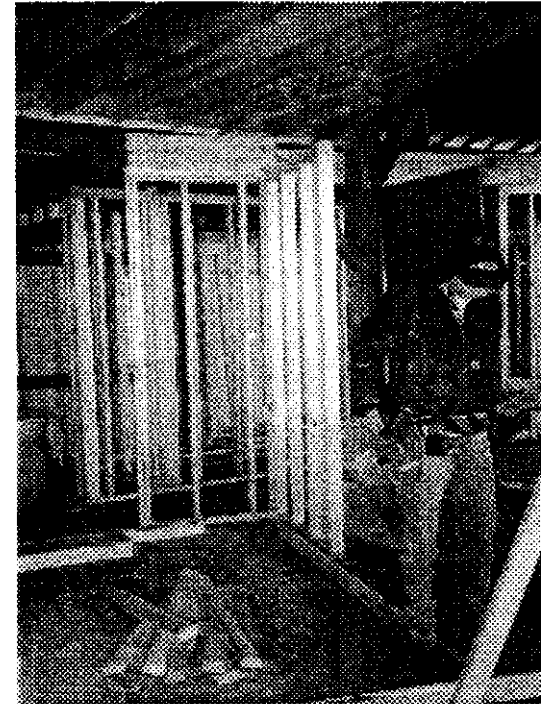
Above: Aaron Haschell reframes the kitchen replacing the corner column with bearing walls.
