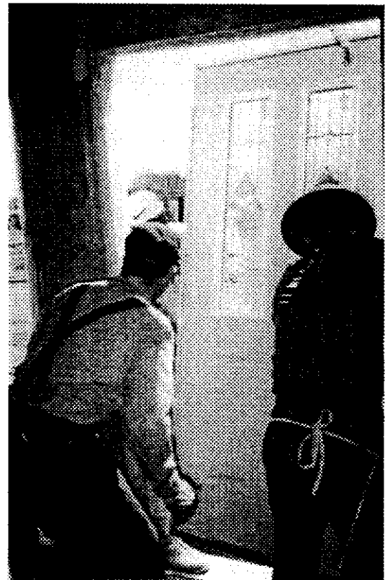
Above: Tony (left) and one of the Amish (right) help to install one of the southern exterior doors.
