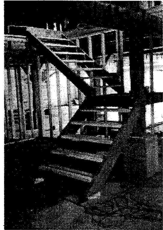
The new stair to the lower level is in place. Due to lack of proper headroom, the original design of the angled stair was abandoned (at the owner's request) and was instead built parallel to the stair above. It does not touch the slab in order to leave room for the brick floor that will be laid at a later date.
