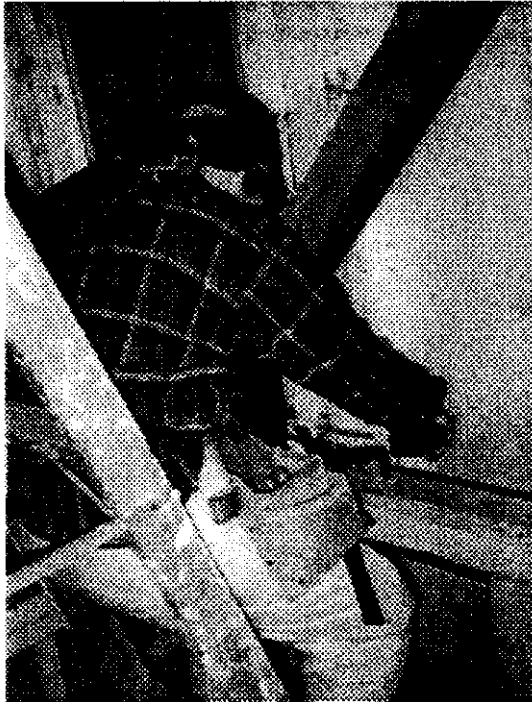
Jeannie Kemble verifies the rough opening of a window in the master bath -- it is being resized.
