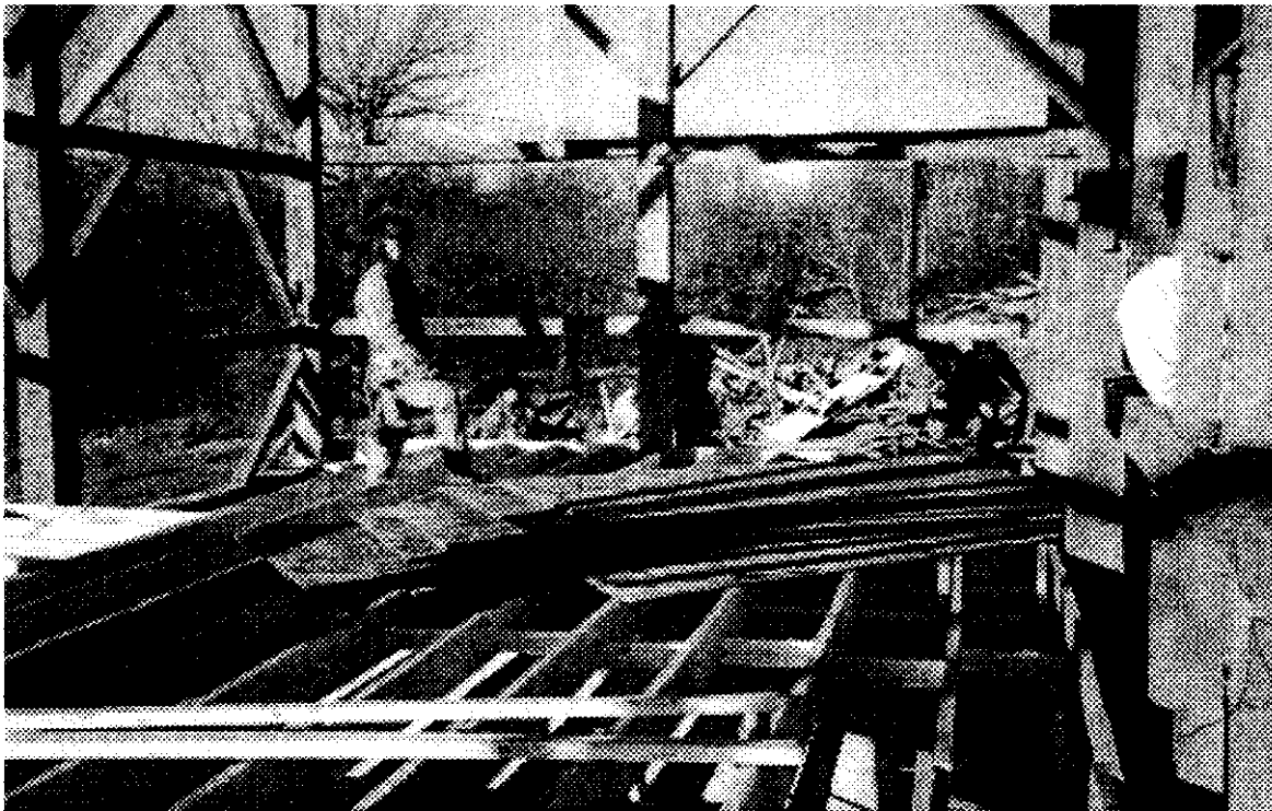
Bob Harmeyer stands in the northwest corner of the main level amidst the new floor joists
