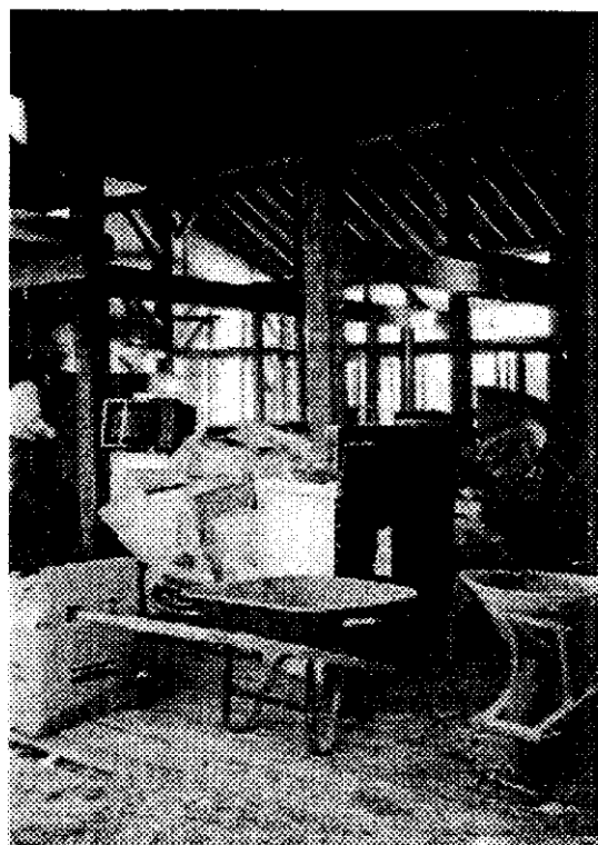
Above: In the beginning much had to be cleared out of the main level in preparation for the new construction.
