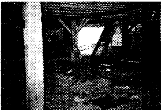
Interior view of existing lower level.
