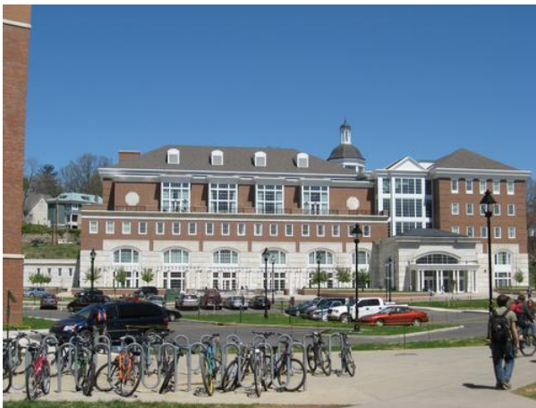
From this view at the back of the building, both the first floor entrance and all five floors can be identified. Copyright 2007 by Ohio University.
